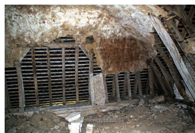
Comble. Phot. Jean-Baptiste Darrasse IVR52_20107200420NUCA
